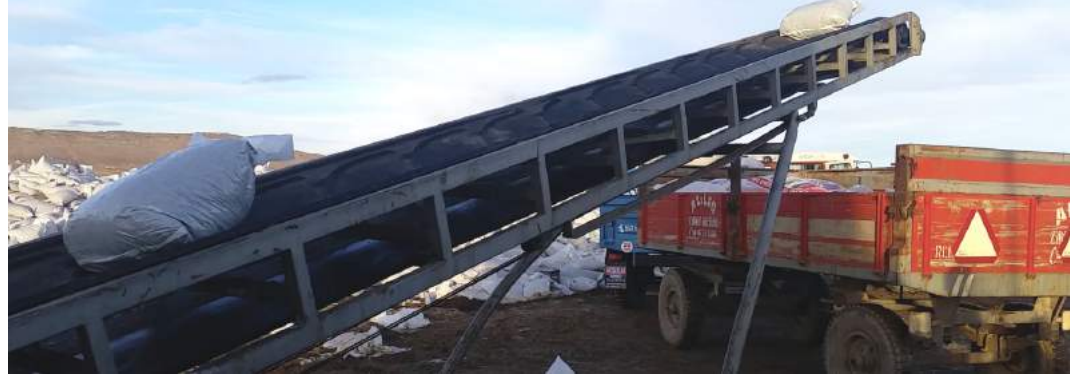
① FEEDER/TRANSPORT CONVEYOR BAND
